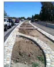
RIVER ROCK COBBLE SET IN CONCRETE
