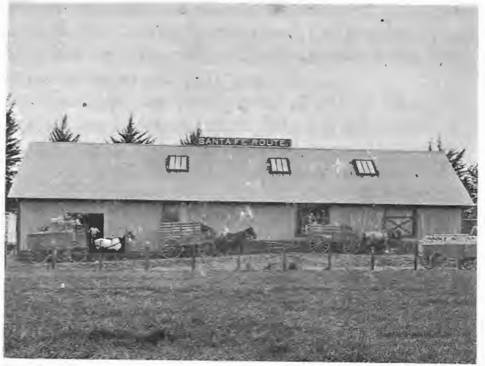
West Duarte Packing House on the Santa Fe between Mountain and Buena Vista. Building not there today. Photos courtesy Duarte Historical Society.
